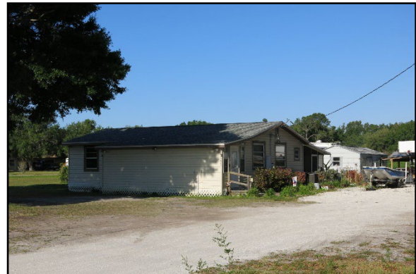
Photo 5.20. 5227 Fort Hamer Road (8MA02617), looking southwest.
