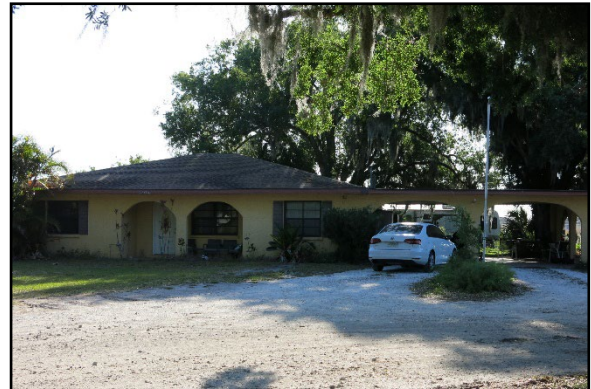
Photo 5.15. 5204 Fort Hamer Road (8MA02615), looking east.
