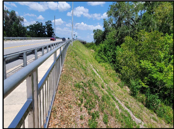
Photo 2.2. Current conditions of 8MA00315 and the surrounding area, facing north.
