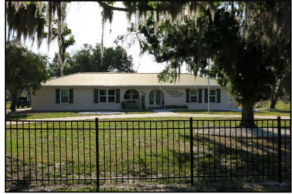
Photo 5.17. 5428 Fort Hamer Road (8MA02618), looking east.
