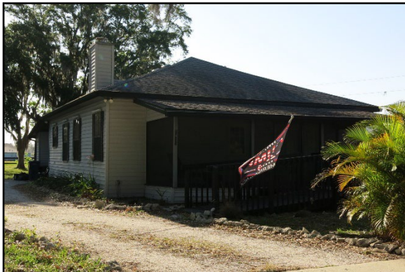
Photo 5.19. 5432 Fort Hamer Road (8MA01216), looking southeast.
