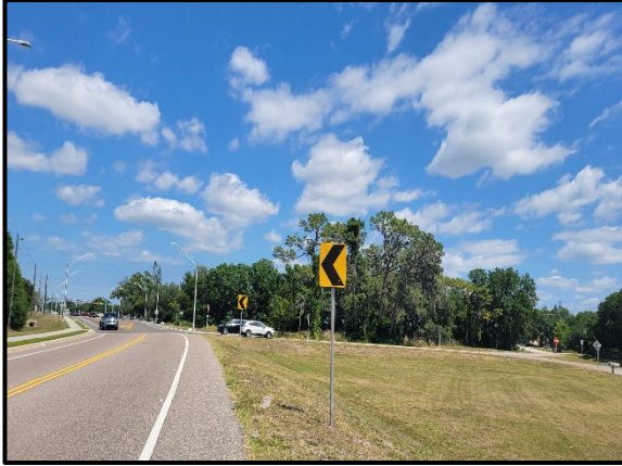
Photo 2.15. View of Fort Hamer interchange and overflow pond toward north end of the corridor, facing north-northeast.
