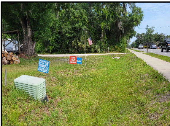
Photo 2.13. Utilities along west side of Fort Hamer Road north of Golf Course Road, facing north.
