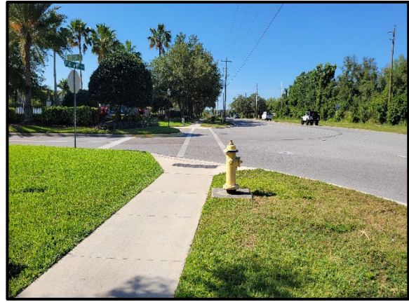
Photo 2.6. Utilities toward Chelsea Oaks on the east side of Fort Hamer Road, facing south.
